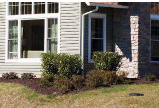
Propane storage can be buried underground with only an inconspicuous service dome showing.
